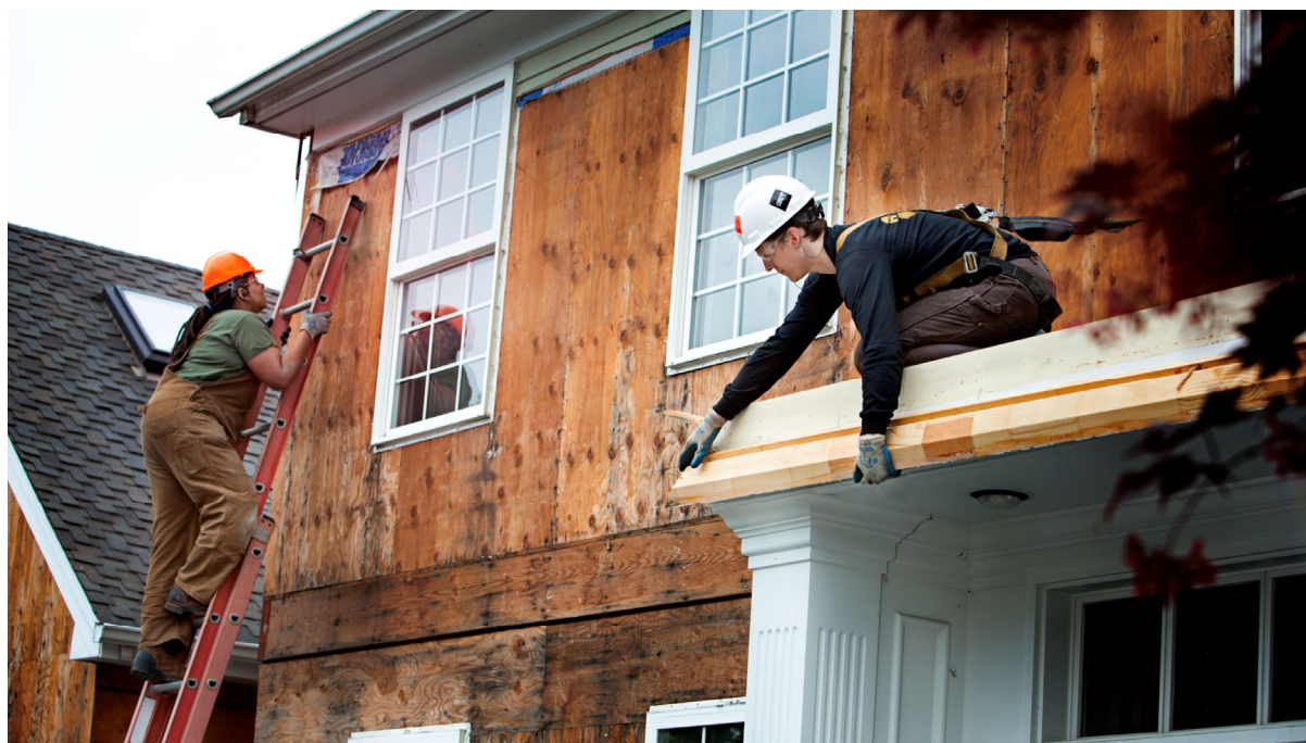
Exterior deconstruction project | Lovett Deconstruction and Salvage Shop
